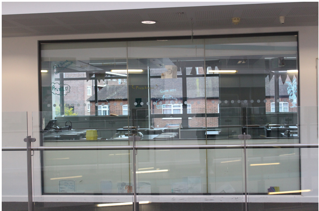
Figure 22 - Windows are placed on both sides of the classroom; windows facing the outside and the corridors beside the atrium
