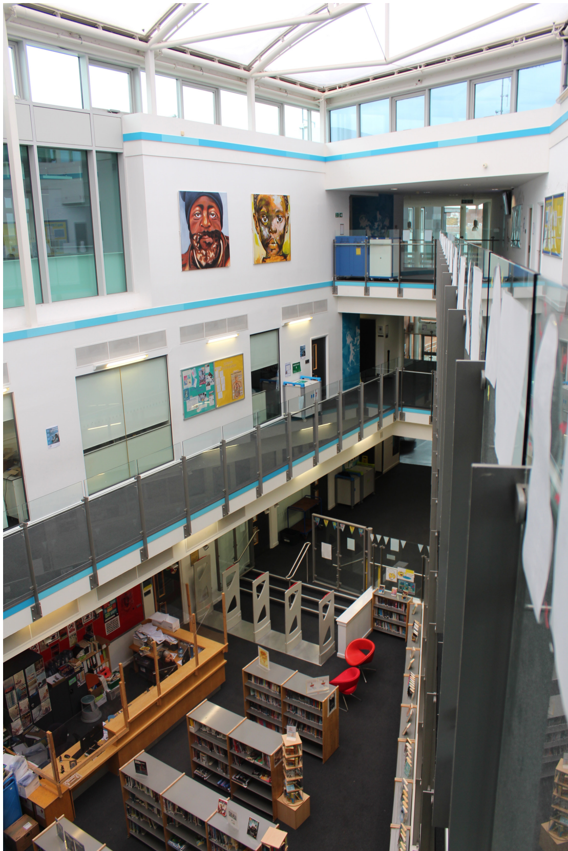
Figure 20 - The 'Bradbury Building' showing the placement of lifts and stairs inside the atrium which consequently disrupts light entering the building and creates dark spaces
